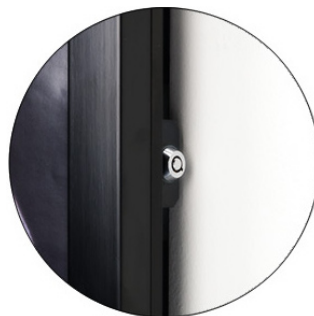
Step 5 Frame is Locked (Stem is Pushed in)
